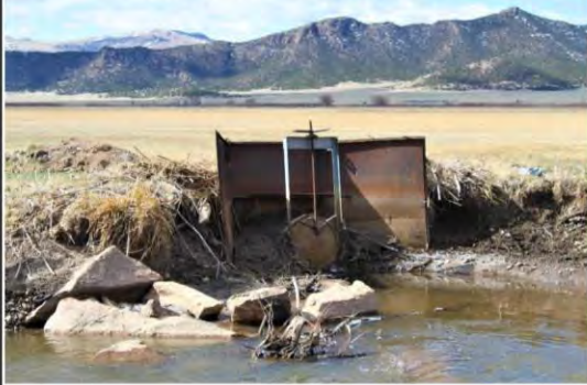
Headgate and diversion dam
