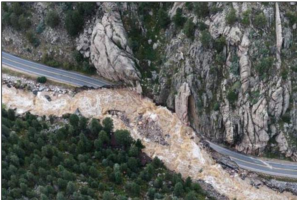
Figure 13. September 2013 Flooding, Highway 34 Big Thompson Canyon, Highway Damage (Photo by Andy Cross, The Denver Post)
