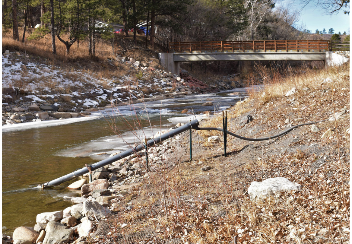
Figure 2. USGS real-time monitoring station with Jasper Road bridge in background.
