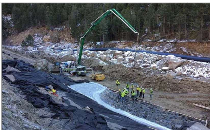
Figure ES-14. Example Image of Repairs to U.S. 34
