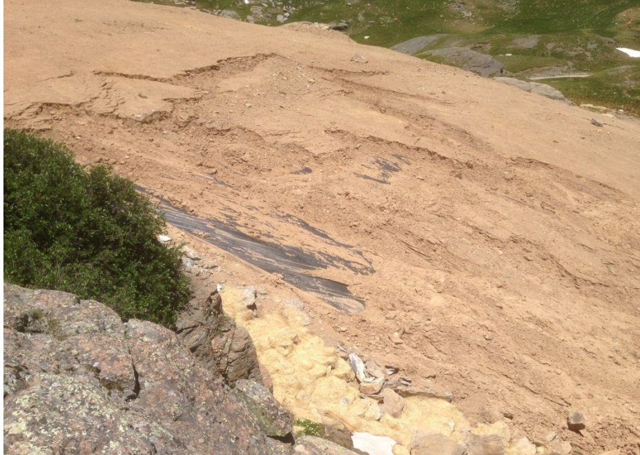
Figure 3 – Soil Slippage – July 2016
