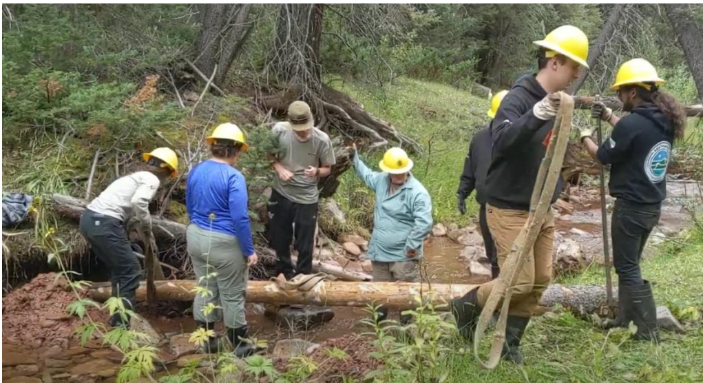
Figure 10 - Installation of the pour-over structures Wildcat Creek Stream-Enhancement Project.
