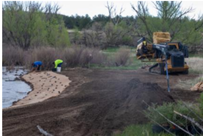
Figure 4 - East Plum Creek bank protections and seeding operation.
