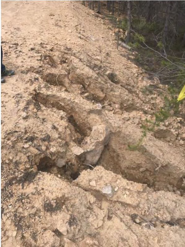
Proposed Log Erosion Barrier (LEB) site #6
