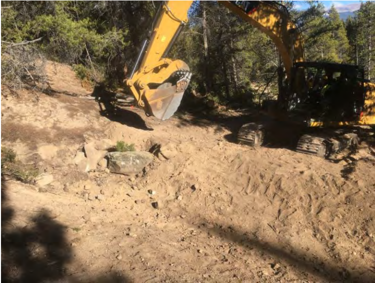
Heavy Equipment Class Building Interceptor Ditch
