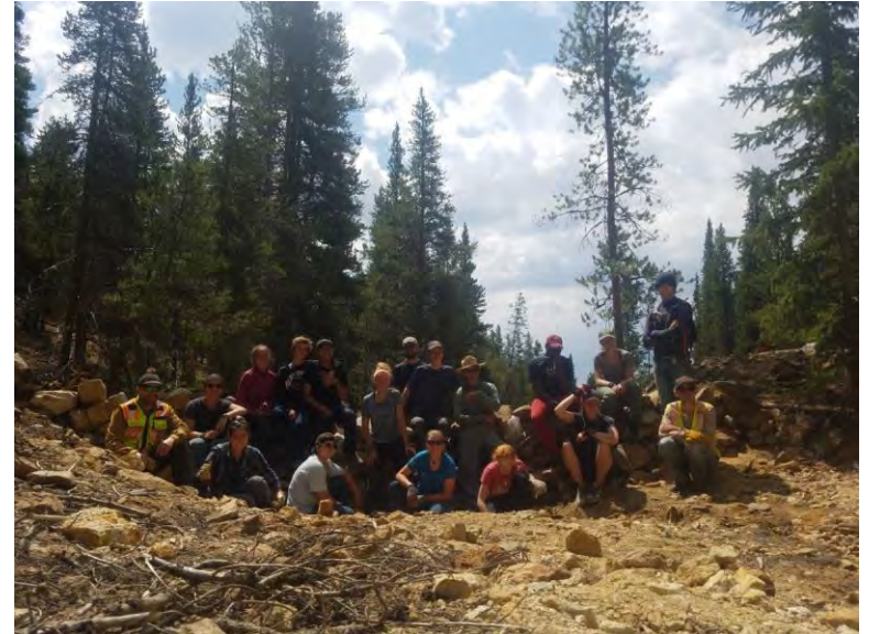
HMI Students Constructing Sediment Basin
