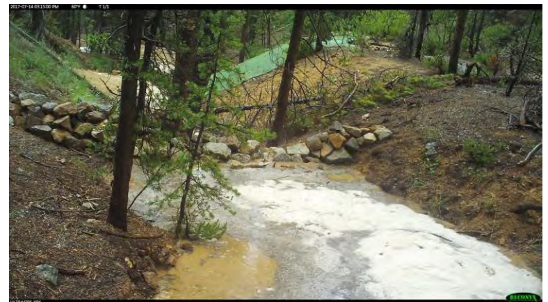
Basin #2 Post-Construction—Rain Event
