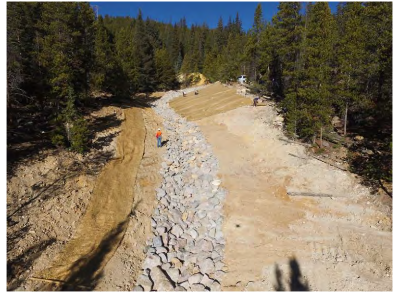
Venture Pile Removed—New Channel Construction
