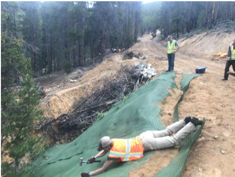
TRM Matting Installation above Little Frying Pan
