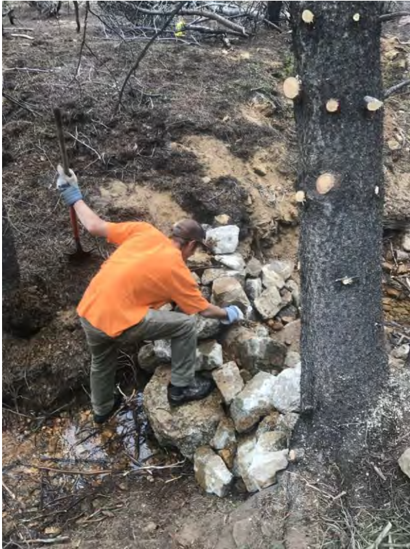
Basin 2 Under Construction
