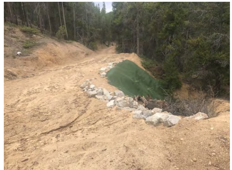
TRM Matting and Stabilization Finalized
