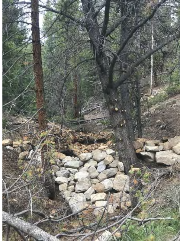
Basin 2 Near Completion, prior to rain events
