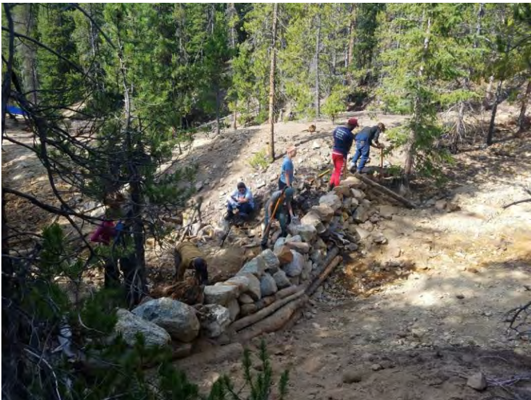
HMI Students Constructing Sediment Basin
