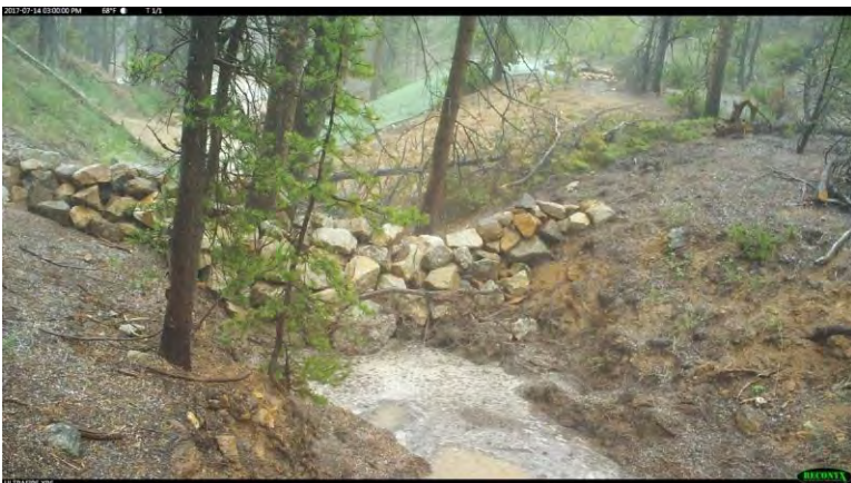
Basin #2 Post-Construction—Rain Event
