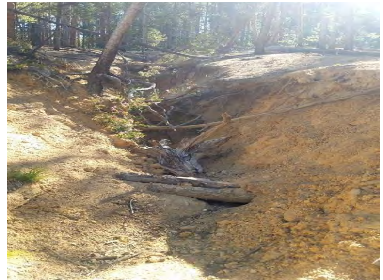
LEB and Channel Roughness Installation Below Powerline Road
