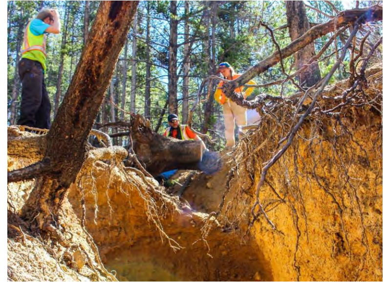
Channel Roughness Modification above Little Frying Pan
