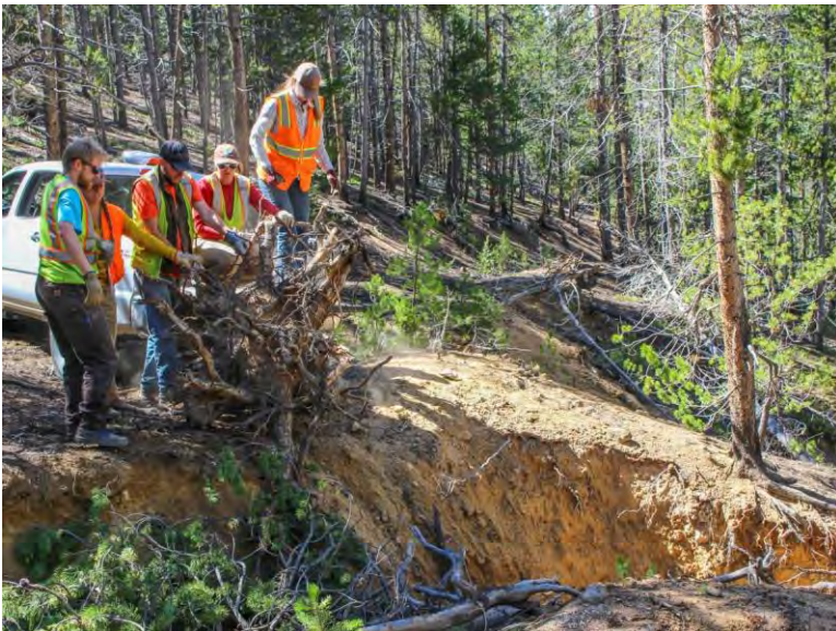
Channel Roughness Modification above Little Frying Pan
