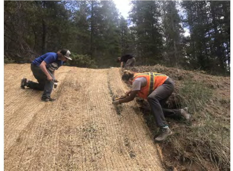
Coconut Husk Matting Installation above Basin #2
