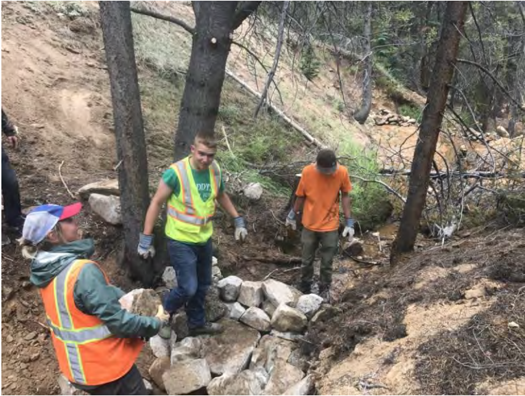
Basin 2 Under Construction
