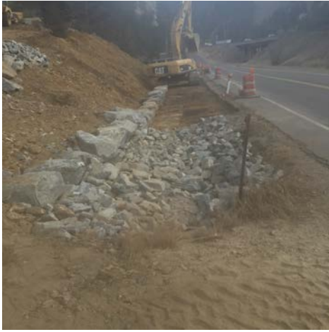
Grading Hoosac the sediment pan
