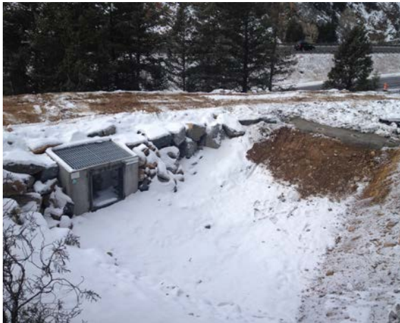
Sediment Basin near outlet of Hoosac Gulch
