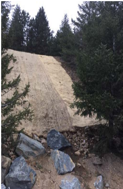
Erosion control blanket on steep abandoned access road
