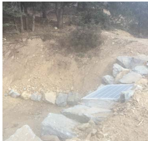
Hoosac Basin Type D inlet structure
