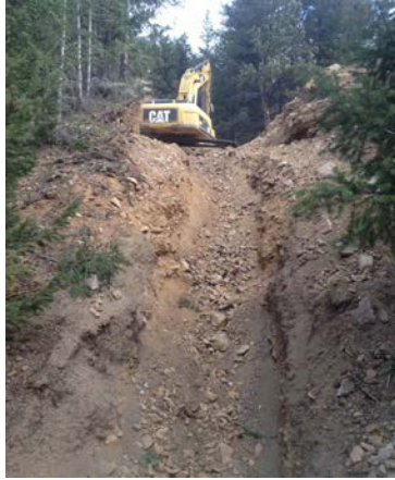
Hoosac Basin Outlet pipe trench
