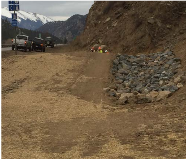
Dumont emergency overflow channel
