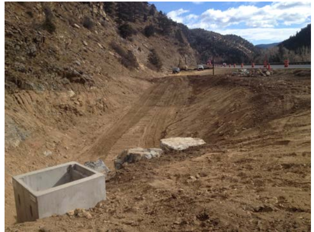
Basin near Dumont on westbound I-70
