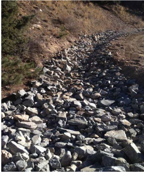
Hoosac emergency overflow channel
