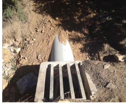
Hoosac outlet pie connection to I-70 cross drain
