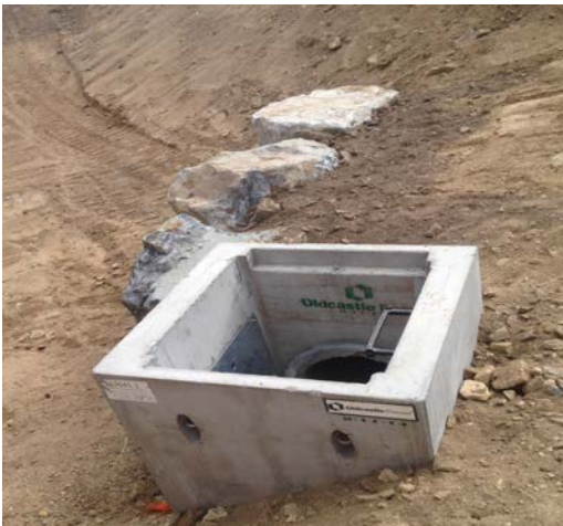
Dumont Basin Type C outlet structure
