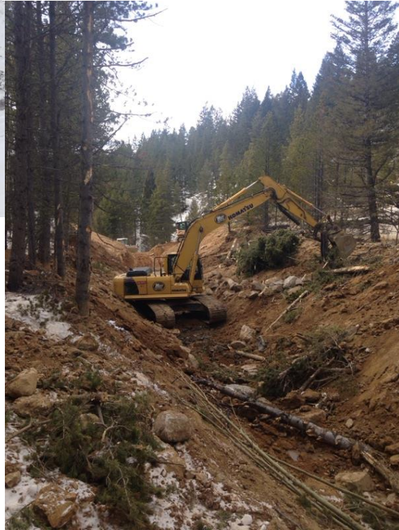
Figure 12 - Large Rock and Grub Placed on Hillside
