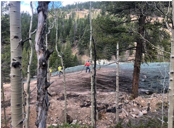
Figure 13 - May 2018 Hydromulch of Repository
