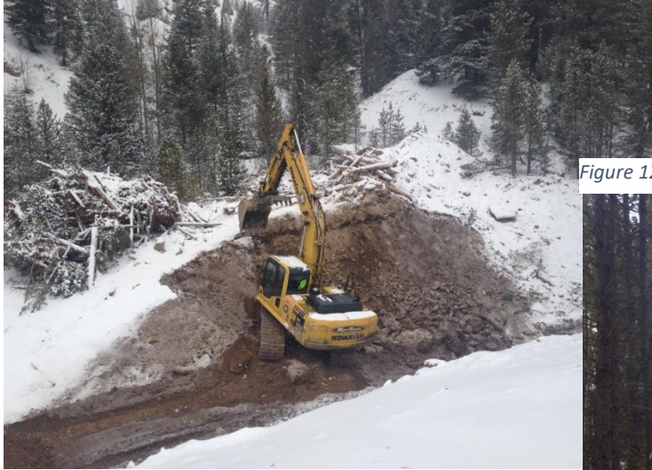
Figure 11 - Dropping Clean Soil Down to Reduce Hillside Gradient
