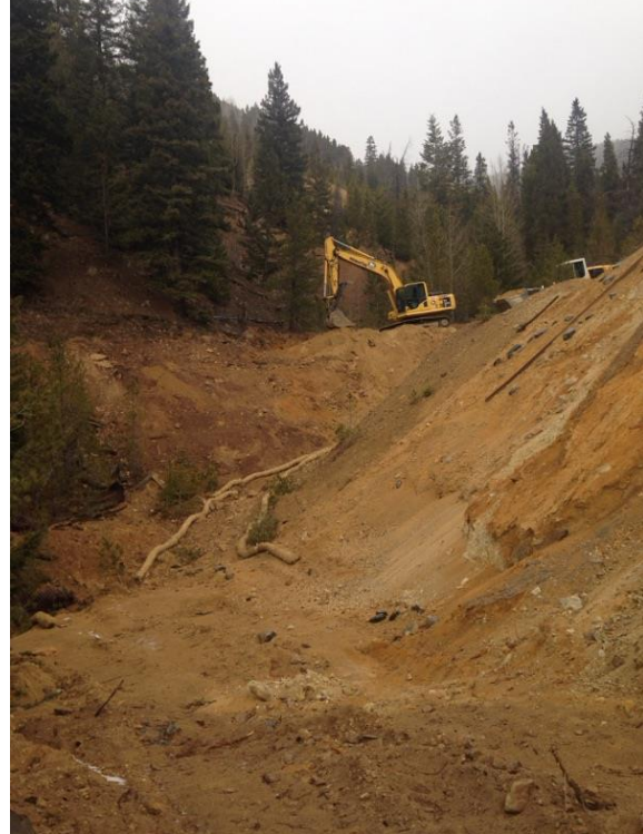
Figure 7 - West Mine Waste Pile Removal Activity
