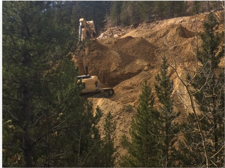
Figure 4 - Equator mine waste pile removal from North Empire Creek
