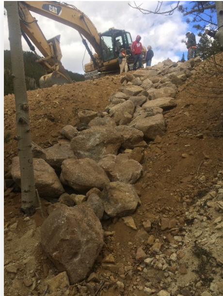
Figure 11 - Rundown Structure for Gold Dirt Run-on control
