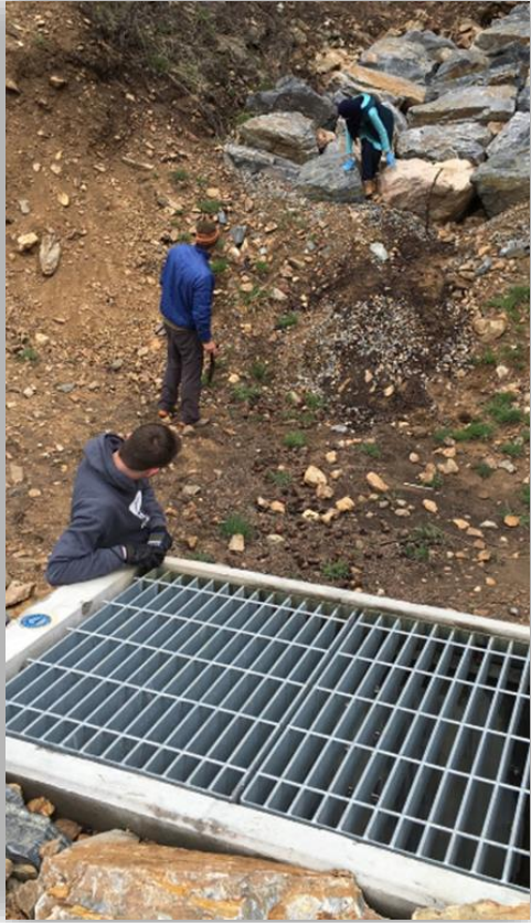
Figure 2 - Water Samples Collected Inside and Outside the Cross-Drain Structure Hoosac Gulch
