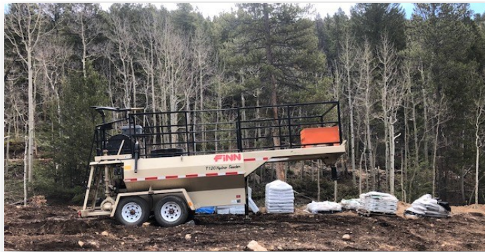
Figure 15 - Staging Area follow-up revegetation effort
