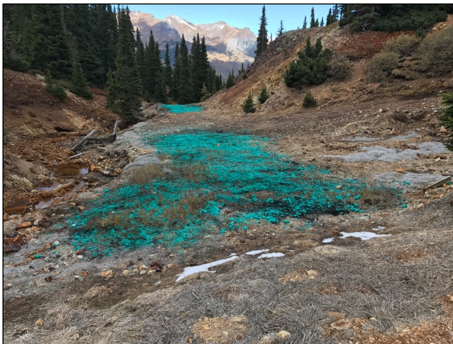
Figure 6. A. Established herbaceous cover in summer 2017 after initial seeding and amendments along Gray Copper Gulch in fall 2015; area excavated of waste rock at Vernon Mine site (downstream view). B. Barren areas were treated with more soil amendments (biochar, mycorrhizal inoculum, and nitrogen fertilizer), seed and hydromulch in fall 2017 (downstream view).
