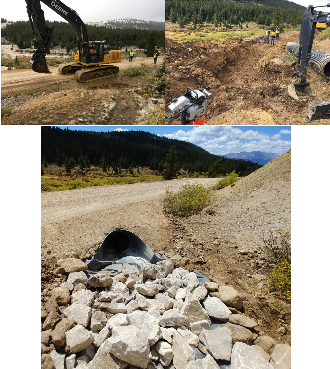
Figure 6.1: Before (upper left) conditions showing excavator and seep flow trending towards the mine waste pile on the edge of the frame and during (upper right) showing depth of excavation and road disturbance necessary to install the culvert. During this excavation, water was diverted around the culvert in the right of the photo. The after conditions (bottom) show installed culvert with collar and interface with lined section of channel. Note that former seep path to the right is dry because water is flowing through culvert in the photo.
