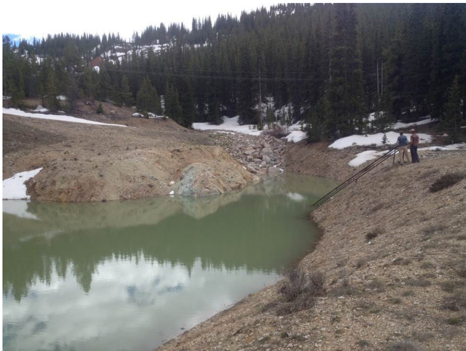
Figure 4.11: Sedimentation pond at the termination of the riprap lined section of Lincoln Gulch.
