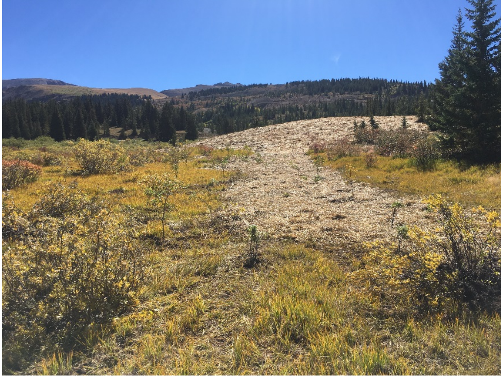
Figure 6.6: (Top) Before conditions showing steep slopes of Valley Mine waste pile along with wetland and dead zone devoid of willow and other species. (Bottom) After conditions showing freshly reshaped pile along with 40 live willow transplants and 100 willow cuttings in the wetland. After amendments were incorporated into the pile, clean fill material was placed on top, seeded, and mulched to promote vegetation growth.
