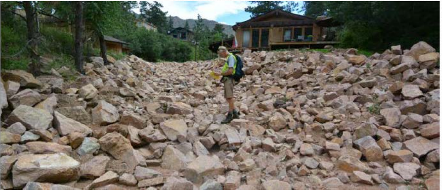
Non-grouted riprap channel
