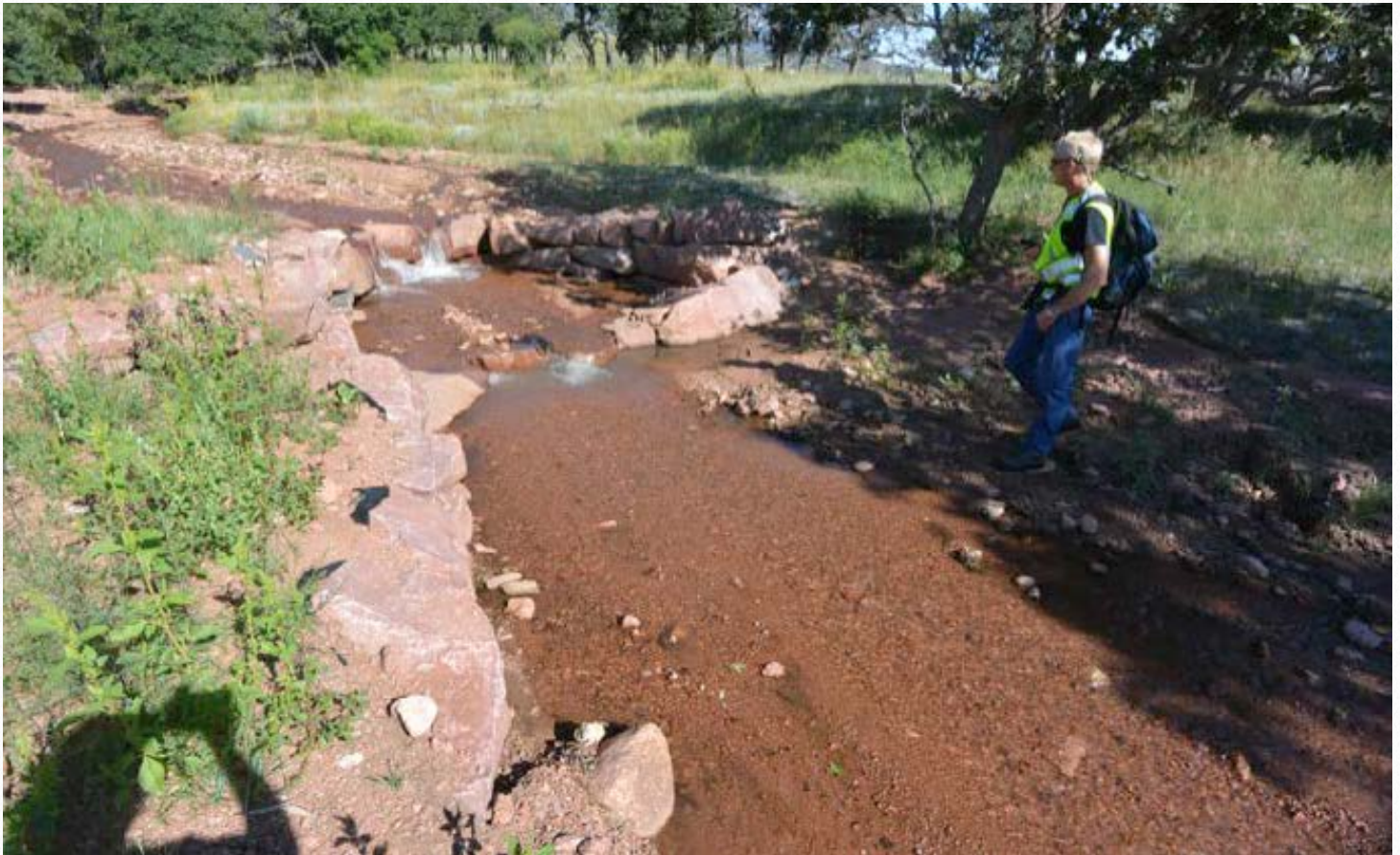
Typical boulder drop structure
