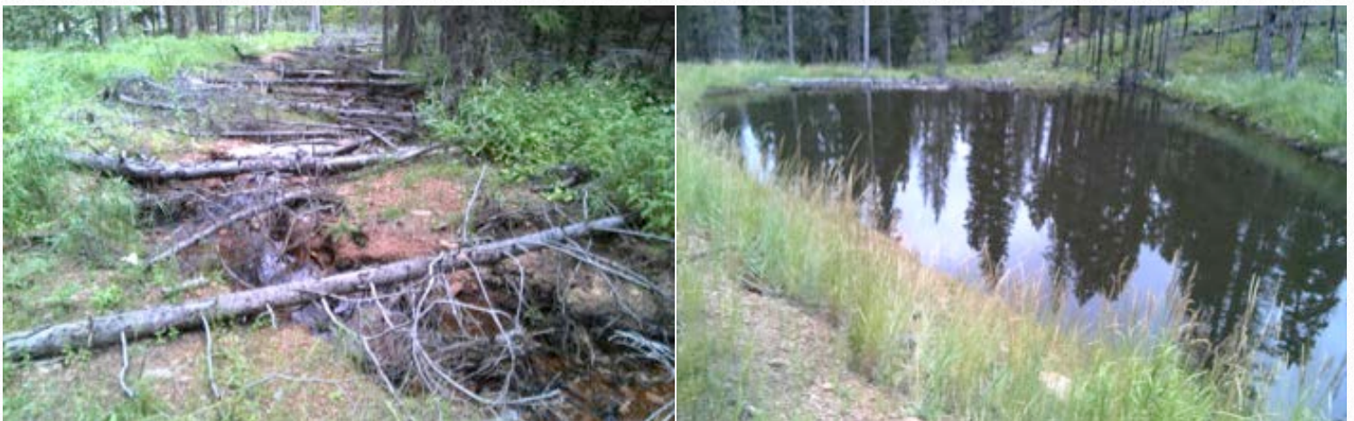
Log corduroy (left) and sediment basin (right)
