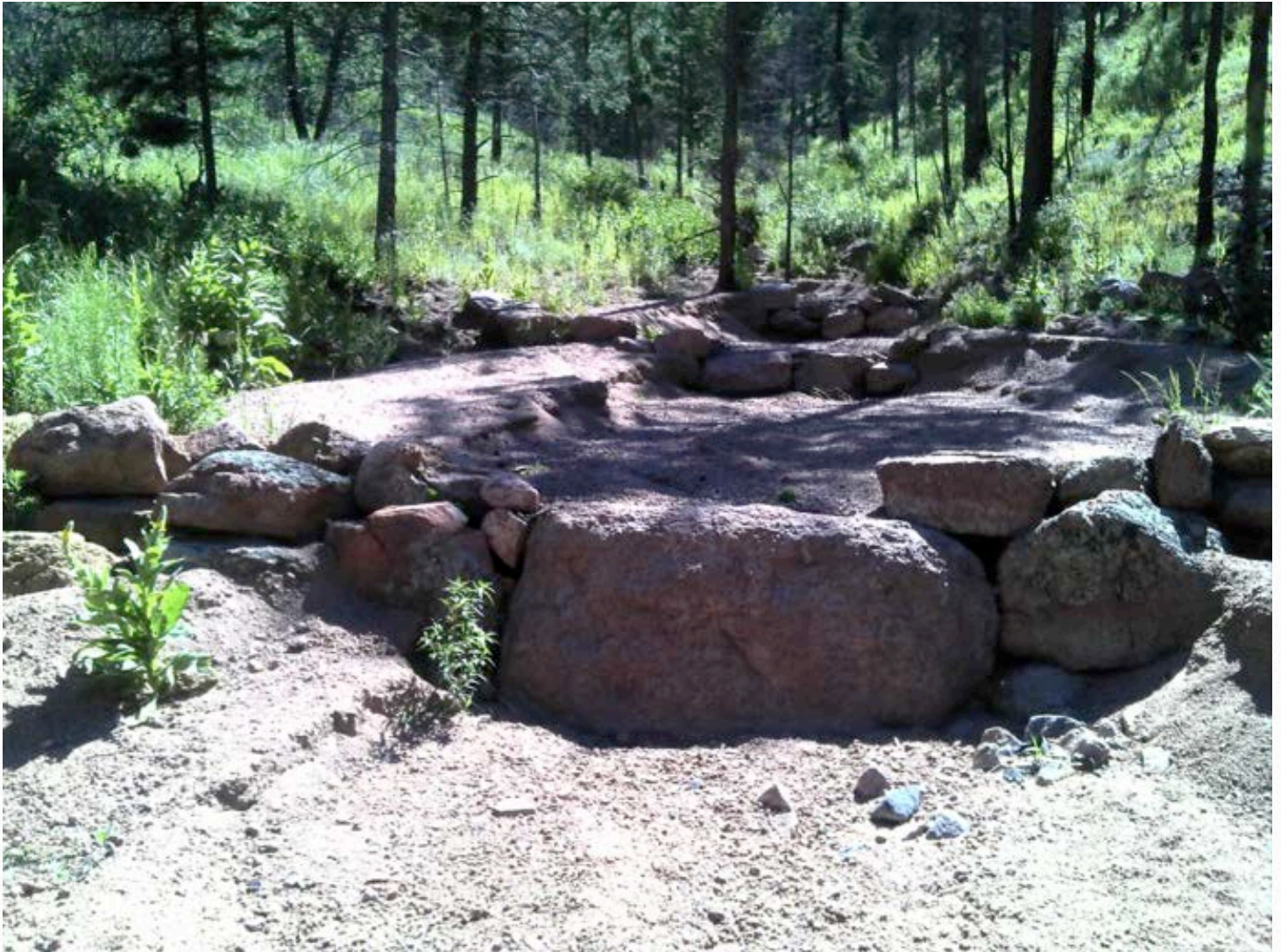
Boulder Drop Structures in Upper Cascade Creek
