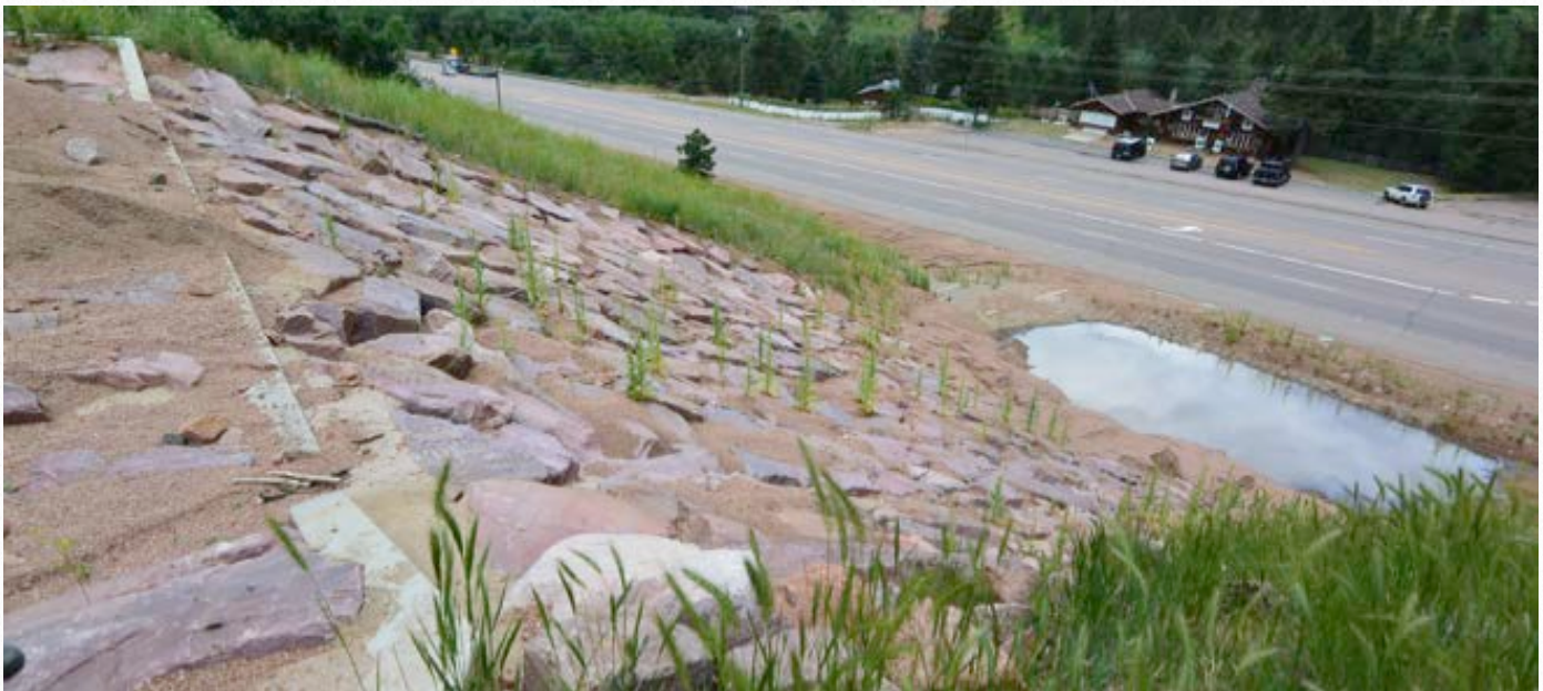
Massive Grouted Boulder Drop Structure & Basin at Spring Gulch.
