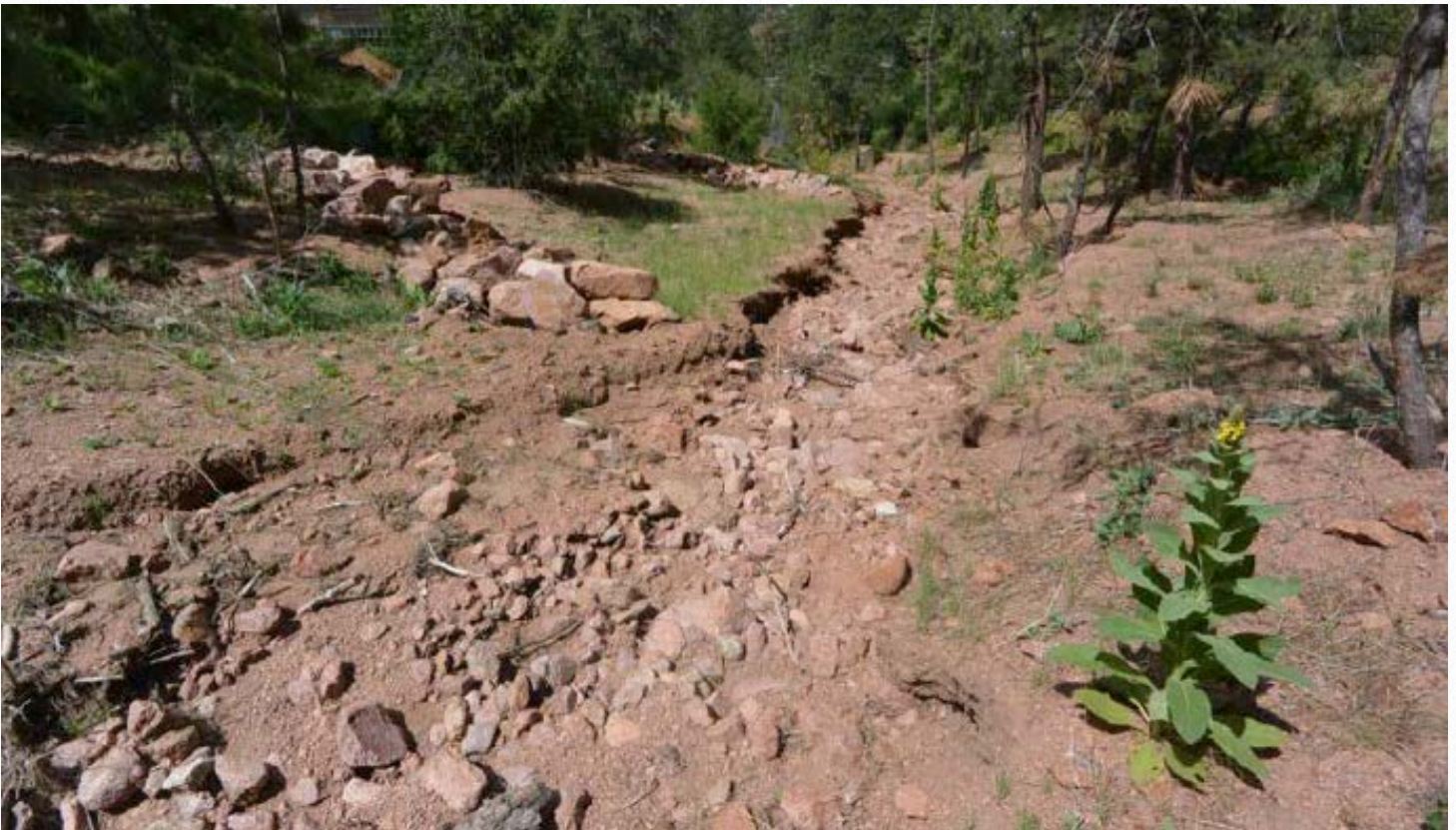
Failed, bendway weir
