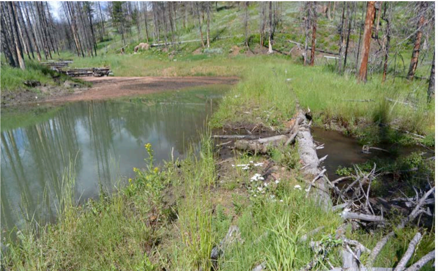
Functioning basin sills in Northfield
