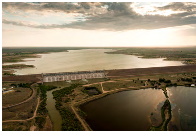
Figure 16: Aerial view of John Martin Reservoir and Dam. Photo courtesy of Bill Cotton, Colorado State University.
